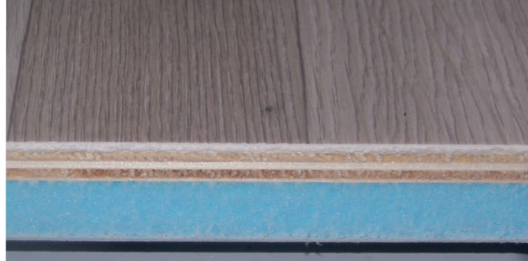
ISOLATION PLANCHER 25MM STYROFOAM
