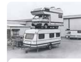
1978 — The innovative PUAL body shell is developed and proves its stability.
