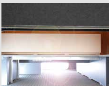
⊕ FRANKIA double floor – stepless and heated with a continuous height of 35 cm
