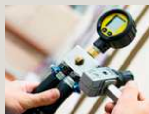
GAS SYSTEM The gas system is pressure tested.
