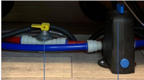
1 – Manual drain valve (hot water) 2 – Frost Control valve (cold water)
