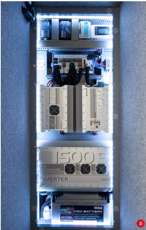
a BÜTTNER ELECTRONIK - comprehensive technology package b 72-cell solar module c Dometic Freshlight (option) - roof air conditioning and skylights in one
