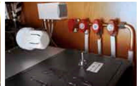
Underfloor heating with shunt
