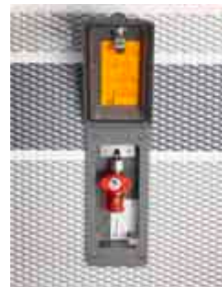
Exterior Calor gas outlet
