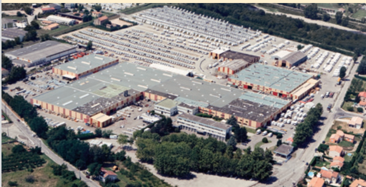
Production site Tournon-sur-Rhône, Ardèche, France
